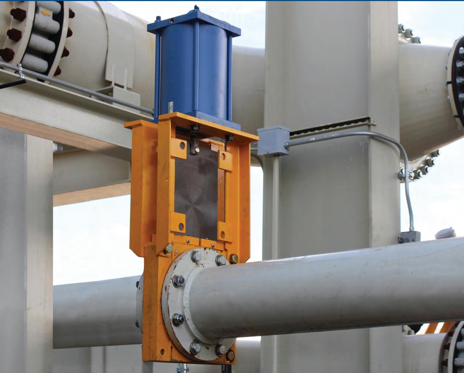
**TGW series valves for slurry applications**
